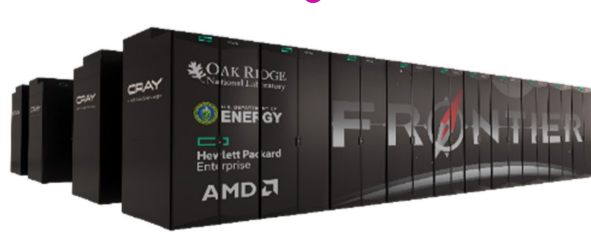
Figure 15. Number 2: Frontier supercomputer at the Oak Ridge Leadership Computing Facility
